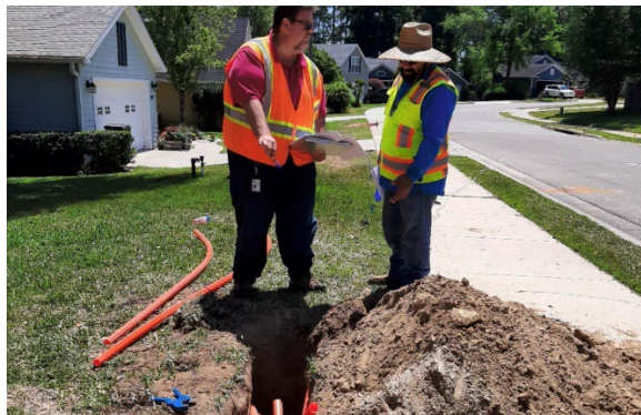
Public Works Continues to Monitor Fiber Installation in County Right of Way
